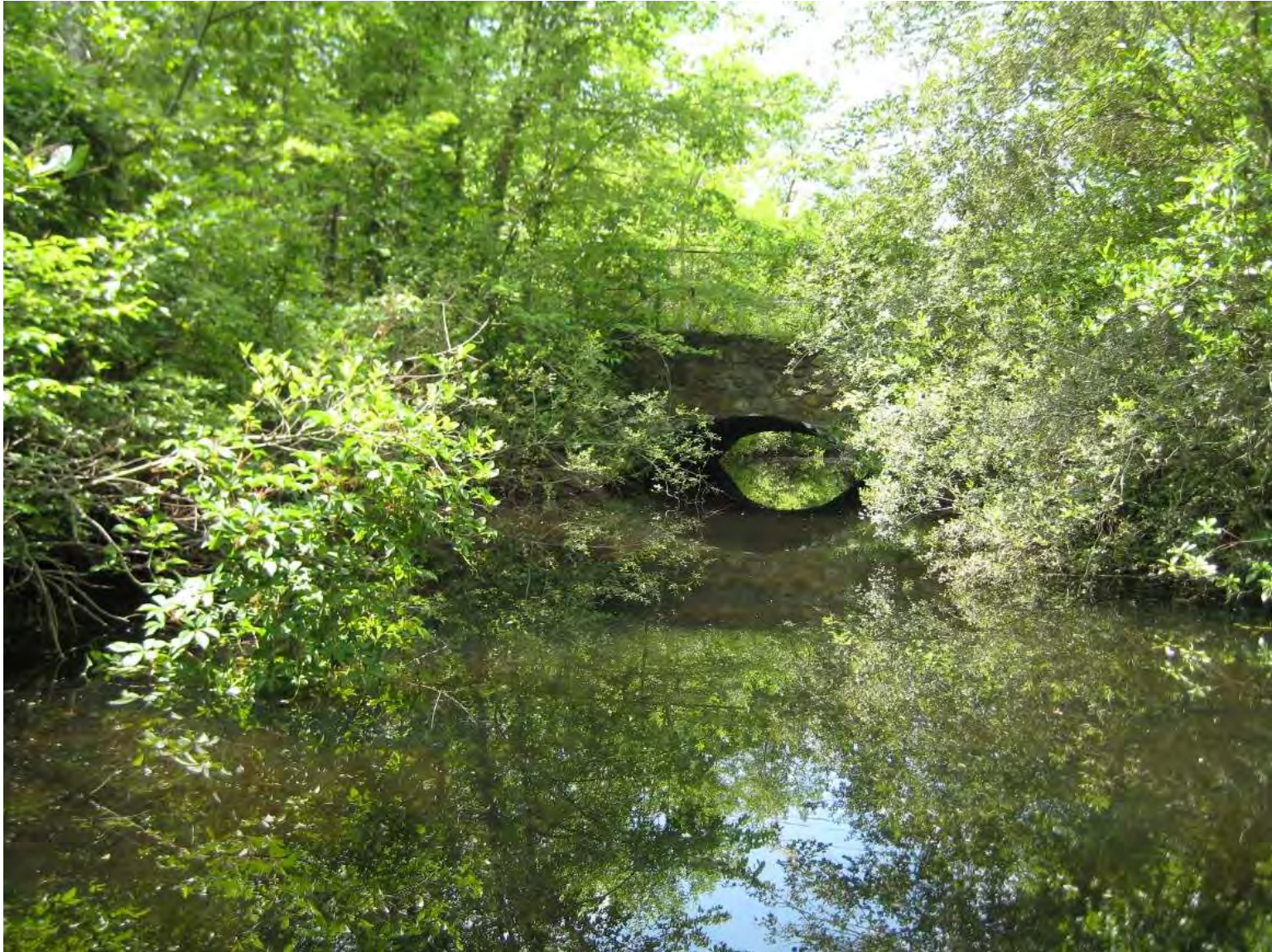
Culvert that was installed c. 1966
