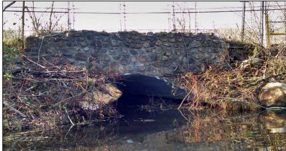
Culvert under Oscaleta Road
