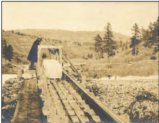
Photos courtesy of Studwell Mead Foundation, Mead Chapel
