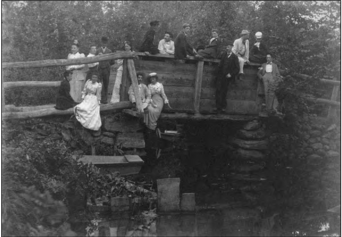
Old bridge over the channel. Photo courtesy of Ken Soltex
