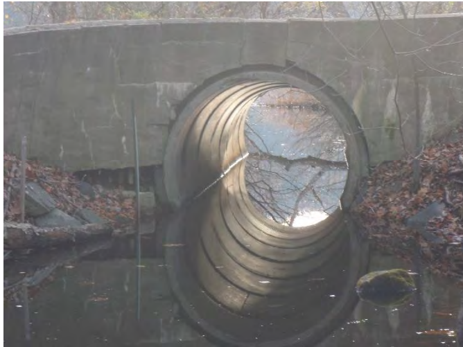
Culvert under Twin Lakes Road
