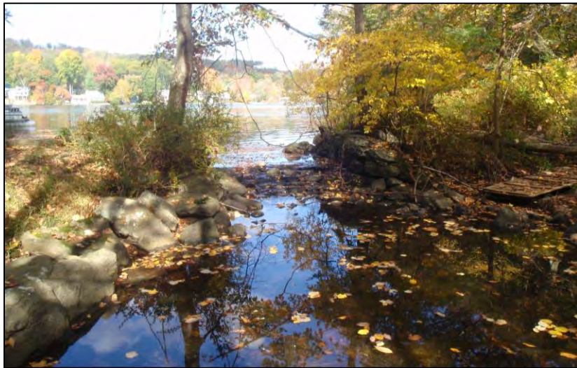
Outlet structure in 2014.
