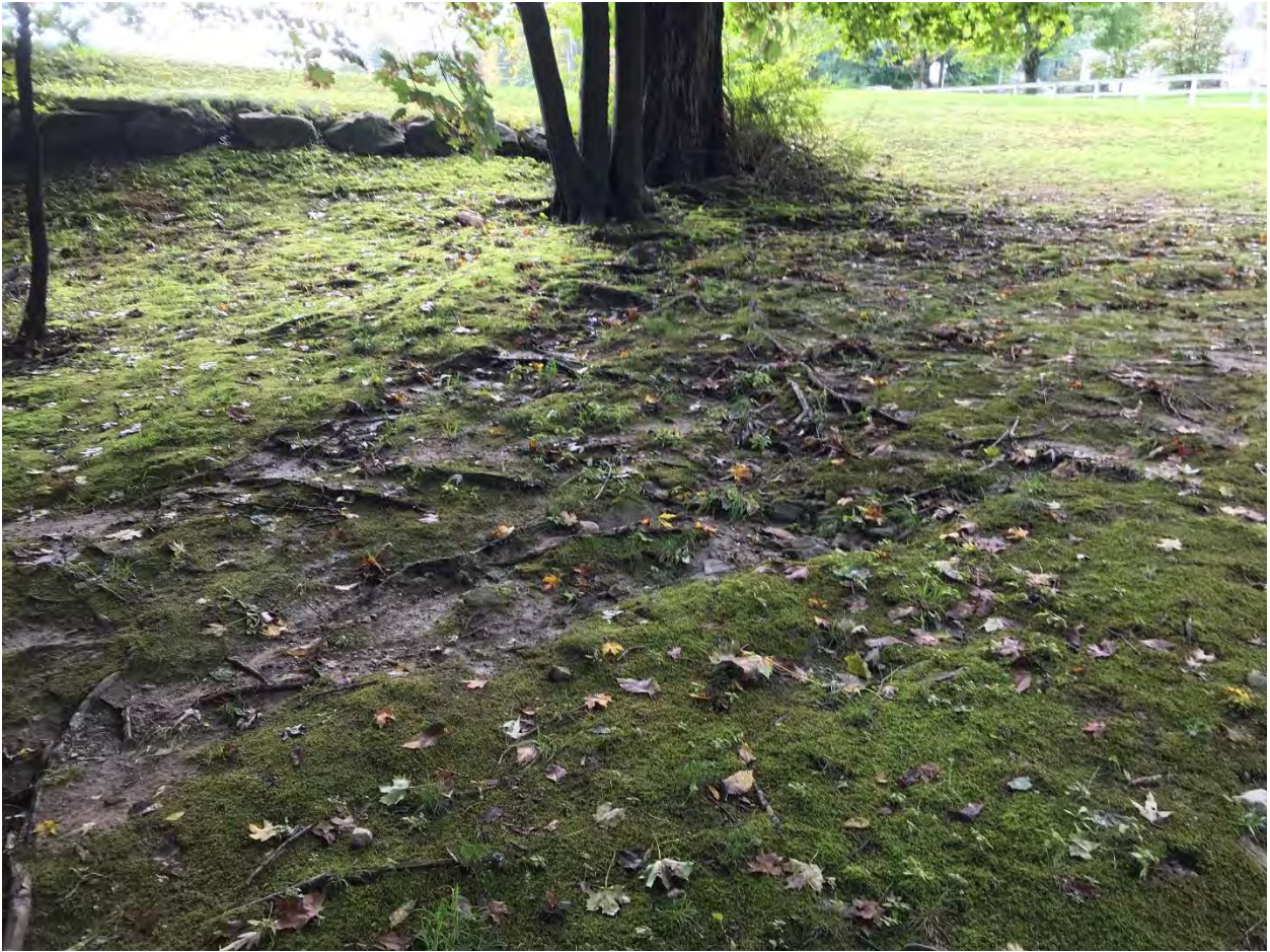
Figure 86 Runoff and erosion from Mead Street into stream (Site 29)
