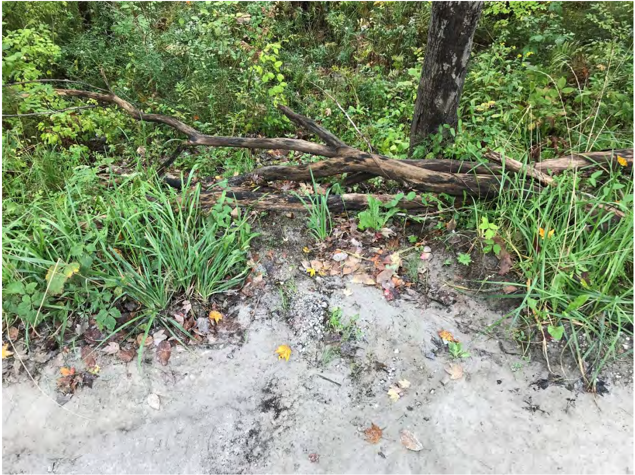
Figure 81 Photo of erosion materials being deposited in wetland and stream on East Ridge Road (Site 28)
